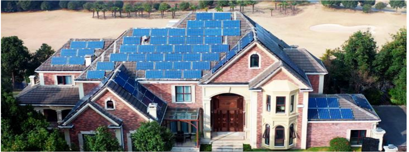
Figure 12. Deploying SP600S Optimizers on Rooftops in Different Orientations to Maximize Installed Capacity
