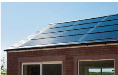
RIDGE TO GUTTER INSTALLATION
