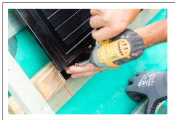
16) Fix panel with 6 screws per panel Don't let the panel drop or slip down as it will not be square
