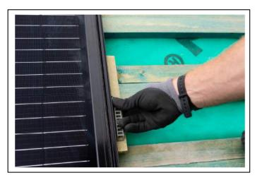
43) Slide panel support into position Parallel with RHS panel frame
