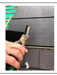
2) Cut off 'leg' if present from RHS internal flashing as surplus to requirements
