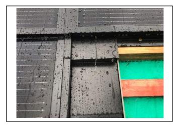
5) Fit internal coupler part 2 under upper Panel to hold in position
