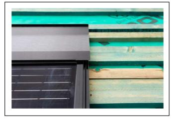
26) When top RHS panel fitted Top flashing will over shoot panel by approx. 30mm
