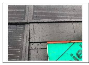
6) Fit bottom flashing Don't forget bottom flashing hooks as standard
