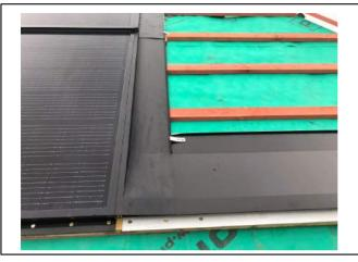
4) Secure with Flashing clip, neoprene washer and screw
