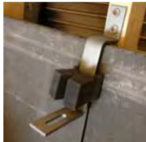
Step 2: Put SolarFlash (small) on the bracket.
