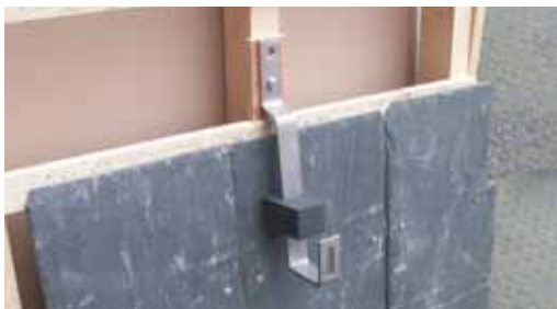
Step 1: Fix foam to bracket drop.
