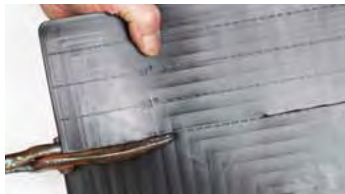
Step 2: As a guide, slate sizes are marked on the SolarFlash.
