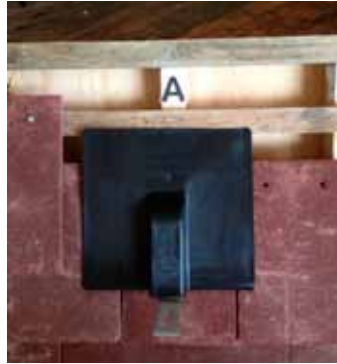
Step 2: Put SolarFlash (small) on the bracket.
