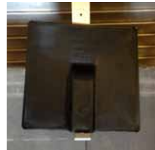
Step 3: Cut tiles around the hood of the SolarFlash as per page 10.
