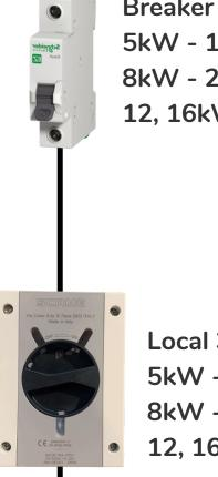
Breaker for heat pump: 5kW - 16A 8kW - 25A 12, 16kW - 32A
