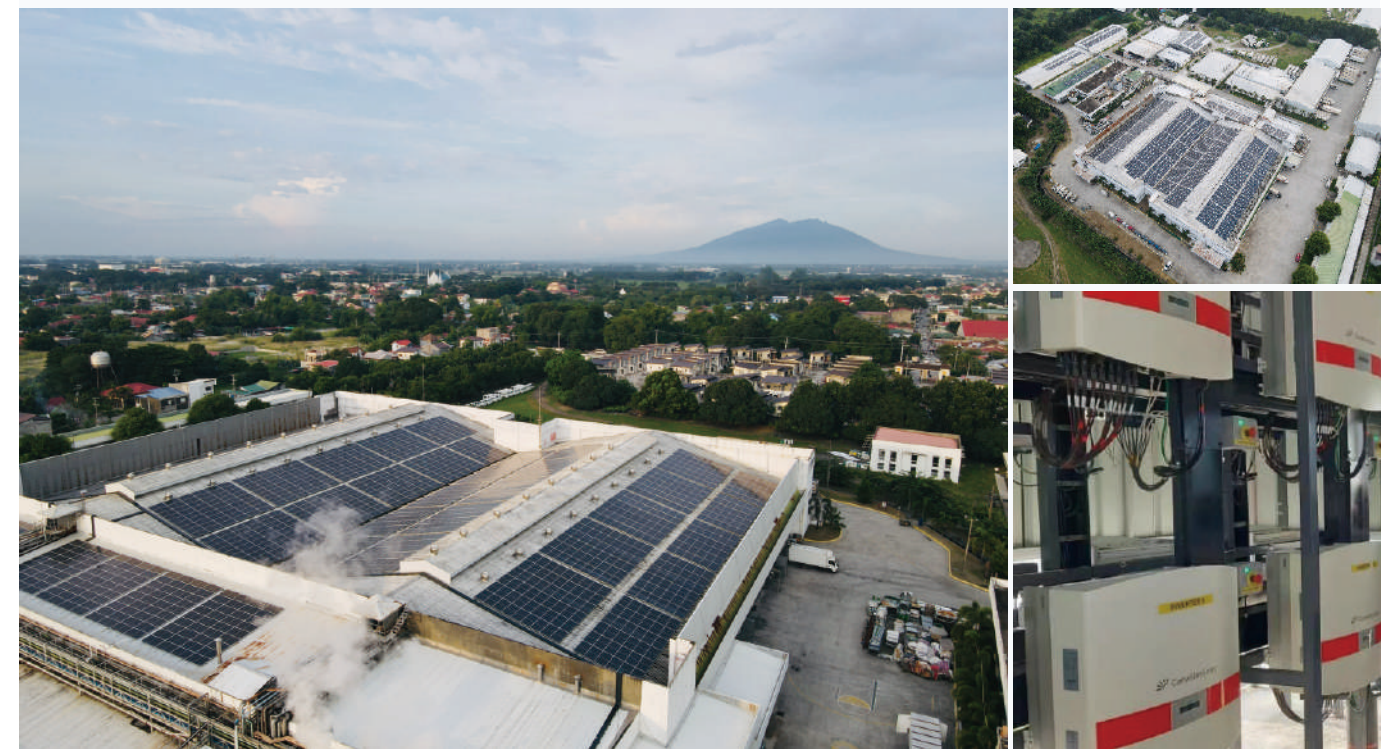
CASE STUDY: Pampanga, Philippines 1.3MW.
