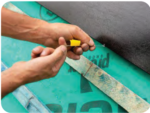
F: Pull flashing hook
