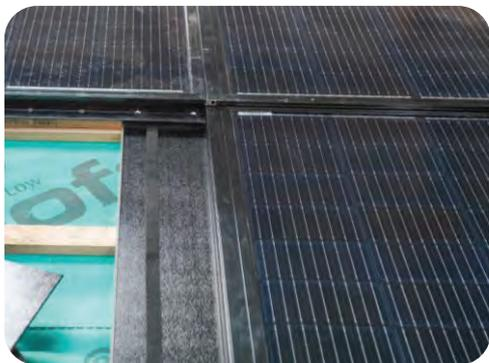
**C:** Fit additional panels around the corner and fit LHS flashing
