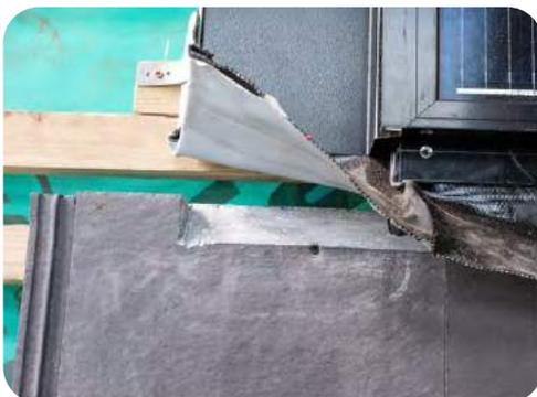
**H:** Grind tile top edge to prevent water pooling
