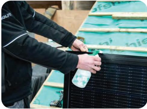
**A:** Use soapy water sprayed or applied to top seal to lubricate & aid fitting
