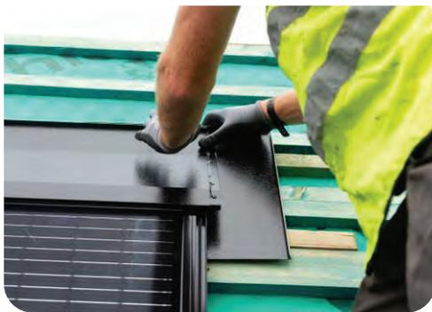
**B:** Insert top RHS corner flashing
