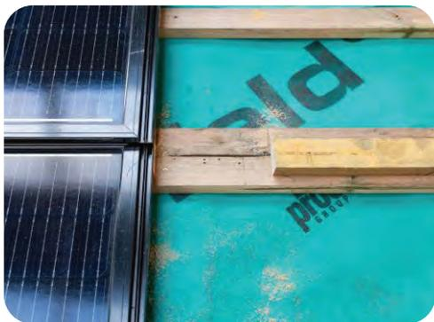
**A:** Cut 170mm section of top batten out from outside RHS edge of panel.
