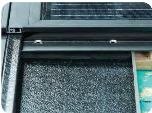
**C:** Fit 150mm section of expandible phone tape under frame of upper panel
