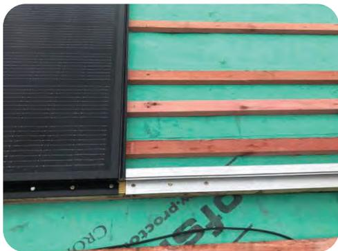
**A: Fit Mounting profile parallel with bottom profile of panel**
