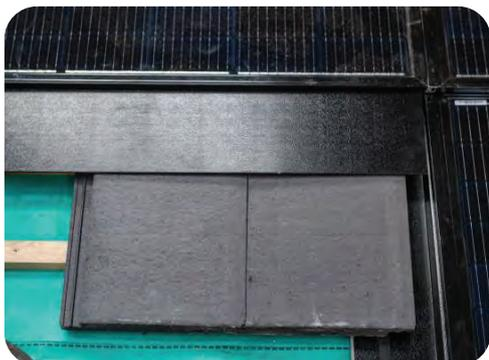
**D:** Fit metal bottom flashing or flexible bottom flashing as standard
