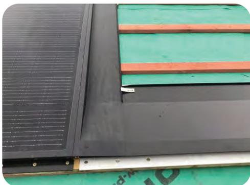
**D: Secure with Flashing clip, neoprene washer and screw**
