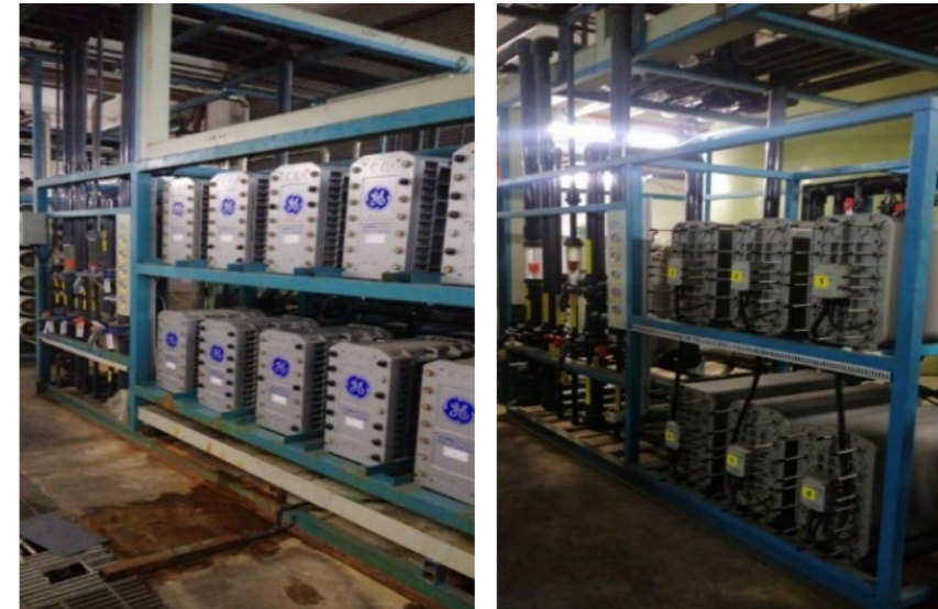
Figure: Optimized EDI system to save water
