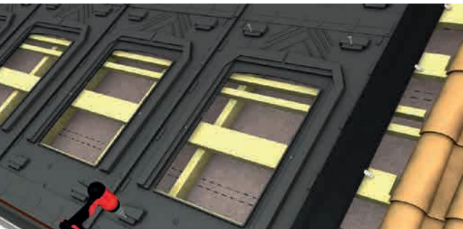
Screwing of GSE supports
