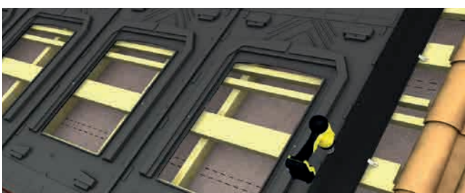
Pre-drilling of GSE frames + flashings + edge wedges
