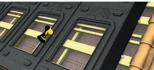
Screwing of GSE frames
