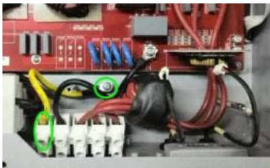
Fig.4.1.2 Inside earth connection
