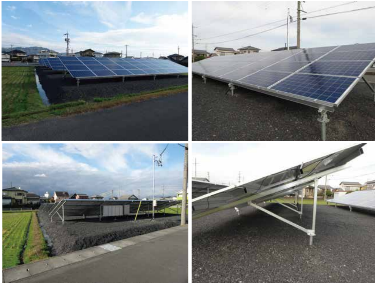
AG4 + Ground Screw, Pile Machine
