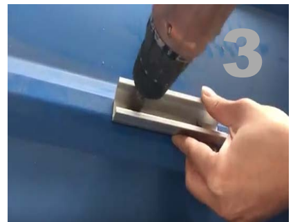
Fasten the mini rail with metal sheet roof with 2pcs st6.3*25 tapping screw.
