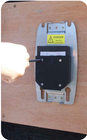
Unscrew the cover on the benector.
