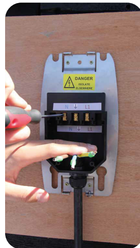
Unscrew the 6 screws (10 screws if installing a 3-phase unit), feed the cable through the gland and secure. Prepare the ends with ferrules.
