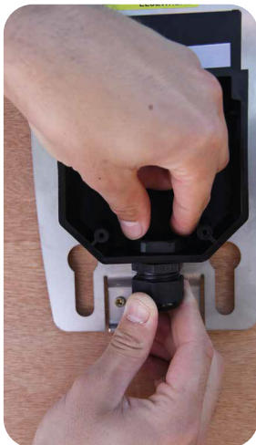
Fit the correct sized gland for your power cable.
