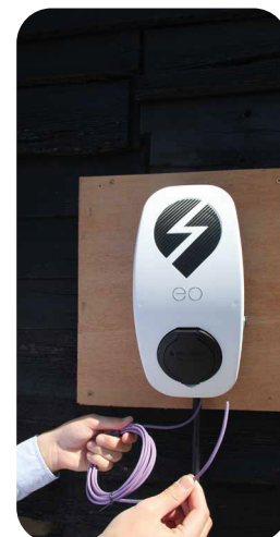
Offer up the charger to the base plate. (If installing an eoGenius ensure that the data cable does not get trapped).
