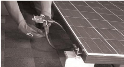
9. Attach the connector clip onto the underside of the module frame.
