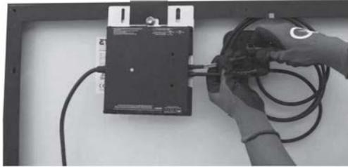
**⚠ CAUTION:** When installing the Engage Cable, secure any loose cable to minimize tripping hazard.
