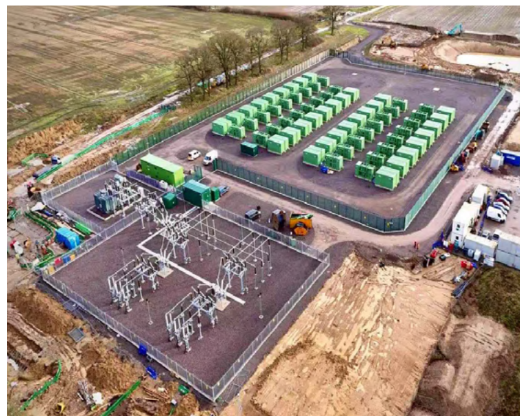
The largest unsubsidized grid-connected standalone battery storage plant in Europe: 100 MW /330 MWh Energy Storage plant at the 400 kV UK national grid substation in Bramley, UK.
