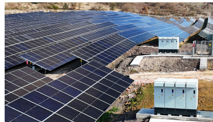
Sixteen x SG4400UD are installed on a foundation base, close to the transformer and MV cabin.
