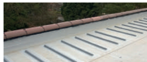
EJObar positioned correctly over membrane strip.
