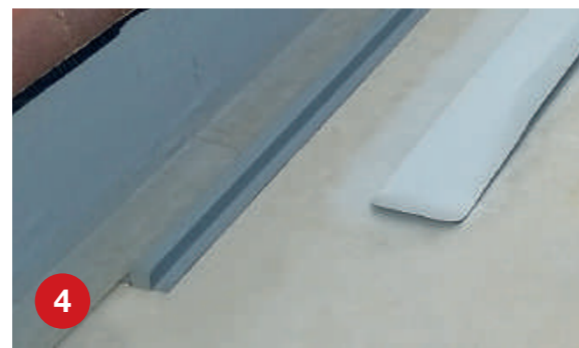
4 Prepare Compatible membrane cover strap, rounding the ends, 100mm longer than the bar.
