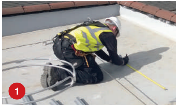
1 Accurately measure and mark out the EJOBAR installation area.
