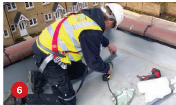
6 Hot-weld EJOBAR in the centre of the reinforced membrane, directly over the line of fasteners.
