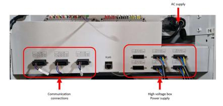
The data connection for metering and PCS can be found under cover 5. Using the cables provided connect the metering and PCS communication cable.
