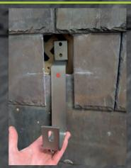
Use shims / packings to create clearance between the bracket and the roofing material.
