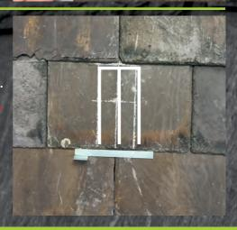
Now you have cut the top slate(s), you need to cut the lower course to create the working area (the area in which the bracket will be fixed).
