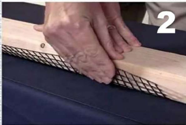
(2) Use a piece of plywood to bend the mesh at a 45-degree angle so that it sits on the roof.
