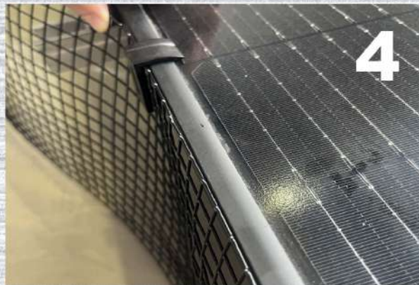
(4) Attach the Fastclips to the side of the solar panel frame and hold the solar mesh securely in place..
