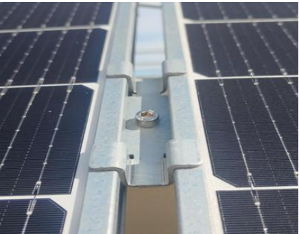
4.On-site photo of the actual installation
