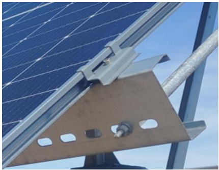
5.On-site photo of the actual installation
